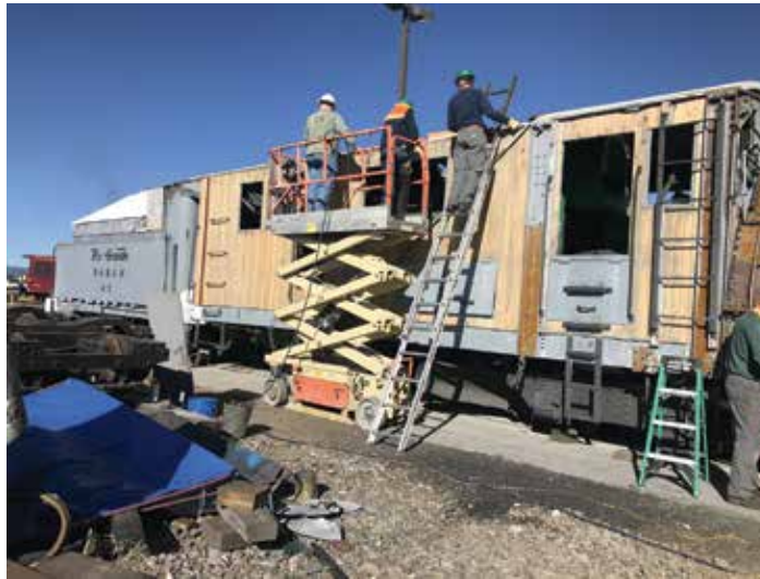
Bryce Templeton, Don Atkinson, and Keith Anderson work on the roof from the scissor lift.
