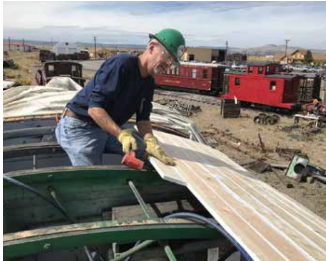
Keith Anderson taps roof boards into place.
