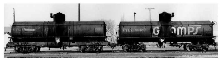
End-to-end, a Narrow Frame UTLX tank car (L) and a Frameless Gramps tank car in Alamosa, December 20, 1952. In 1956 these two cars were renumbered as Narrow Frame 11007 and Frameless 11043. Photo by Robert Richardson. FC&TS Collection, AMP06-118
