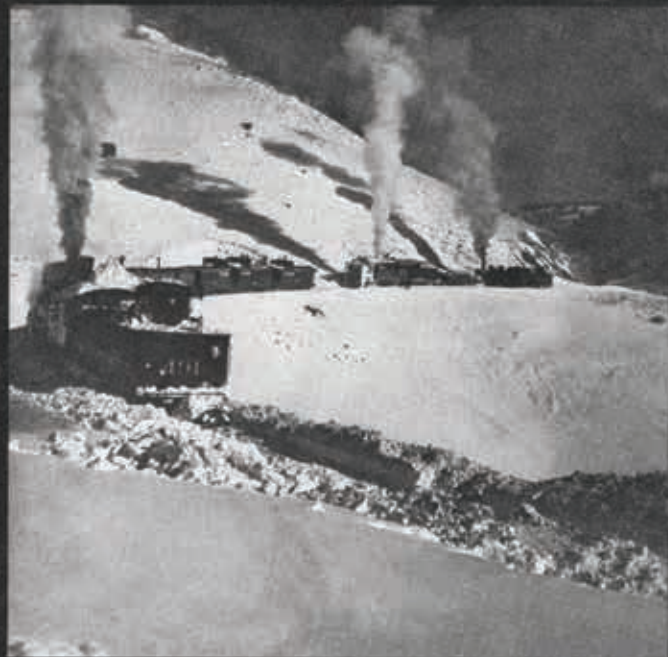
FOLLOWING an unsuccessful attempt to pull out 491 on January 7, workmen built fires under the frozen cylinders. Two mornings later they made another try. The locomotive came out with such ease that the engines jarred the cook car, spilling pork, beans, and cook.
