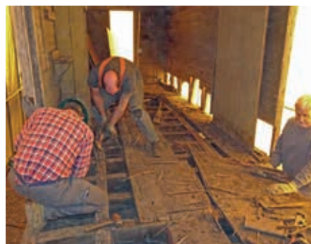
The interior floor was removed which exposed both the frame and original 1881 wood-shaving insulation.
