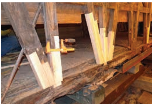
Rotten cross-member framing was replaced as needed at the sill plates.
