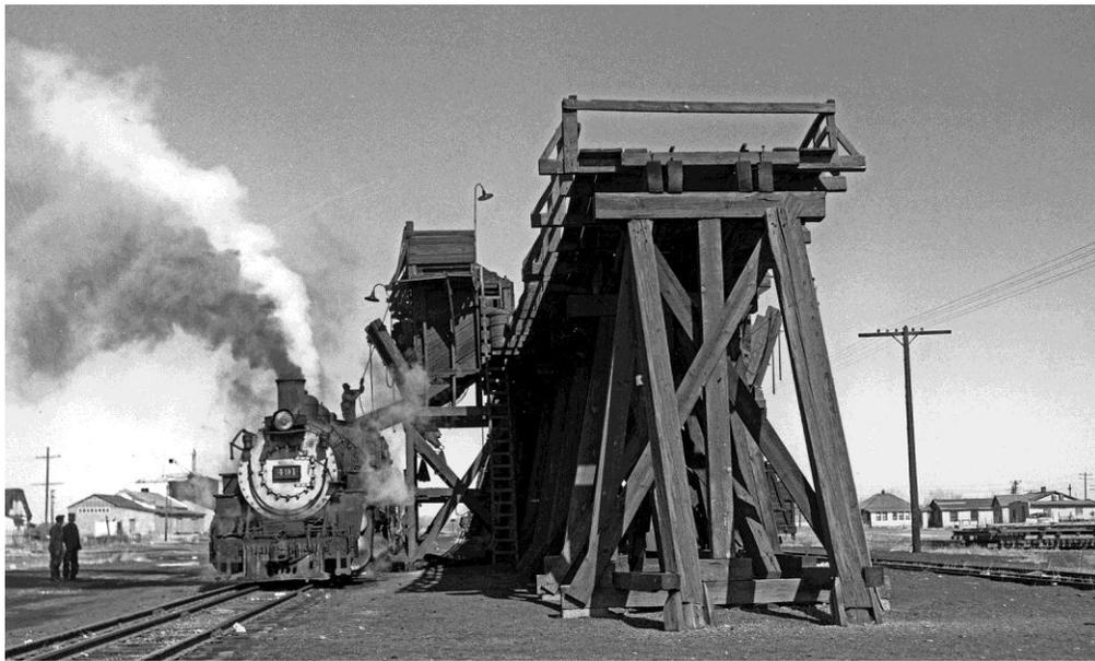
On February 20, 1956, Bob Richardson caught D&RGW K-36 #491's fireman attending to the loading of a tender-full of coal at the Antonito coaling trestle which was replaced by a "Red Devil" coal loader in the late 1950's. There were three elevated bins in this structure, presumably capable of refueling one engine each.
