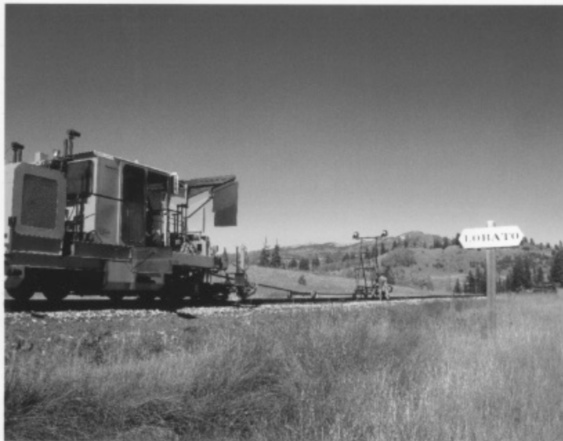
Tamper pushing laser alignment equipment. (Richard Tower)
