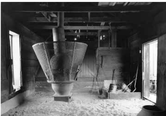
The cyclone tank awaits the crane for final installation.
