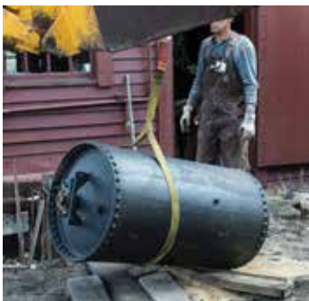
The restored air/sand mixing tank is lowered into its position below the floor of the Sand House
