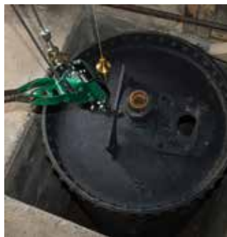
The restored air/sand mixing tank is lowered into its position below the floor of the Sand House
