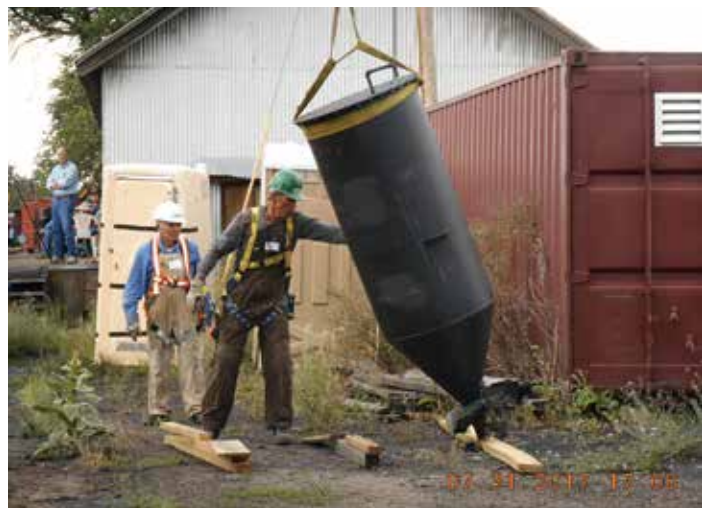
The restored air/sand mixing tank is lowered into its position below the floor of the Sand House
