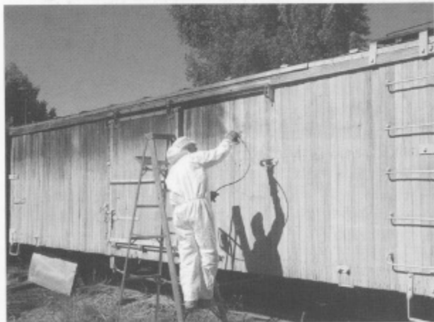
Jerry Hawkins spraying on the oil-based primer coat.
