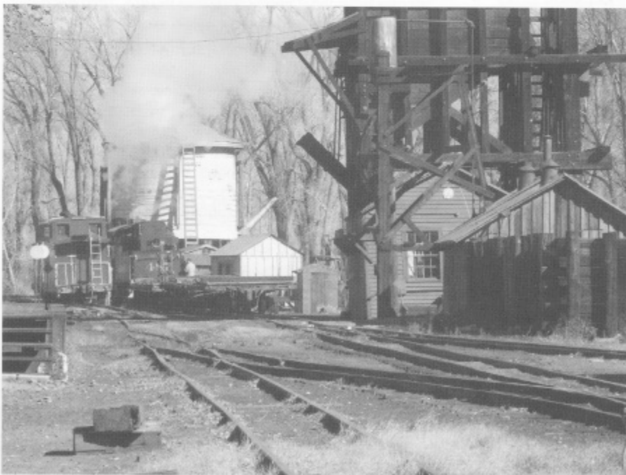
The key facilities for care and feeding of the C&TS steam locomotives are located in this area. The planned RVC will allow visitors to more easily understand the function of each structure and view the activities taking place here. (David Lee)
