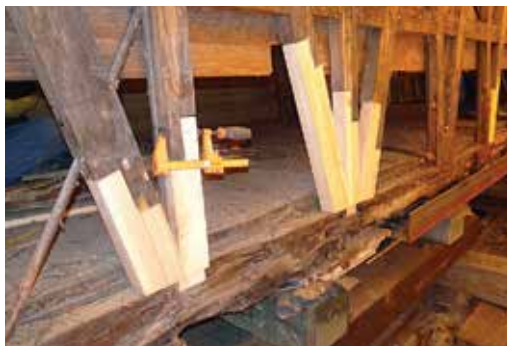
Rotted cross-member framing was replaced as needed at the sill plates.
