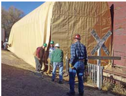
Protection from the elements for both rolling stock and personnel.
