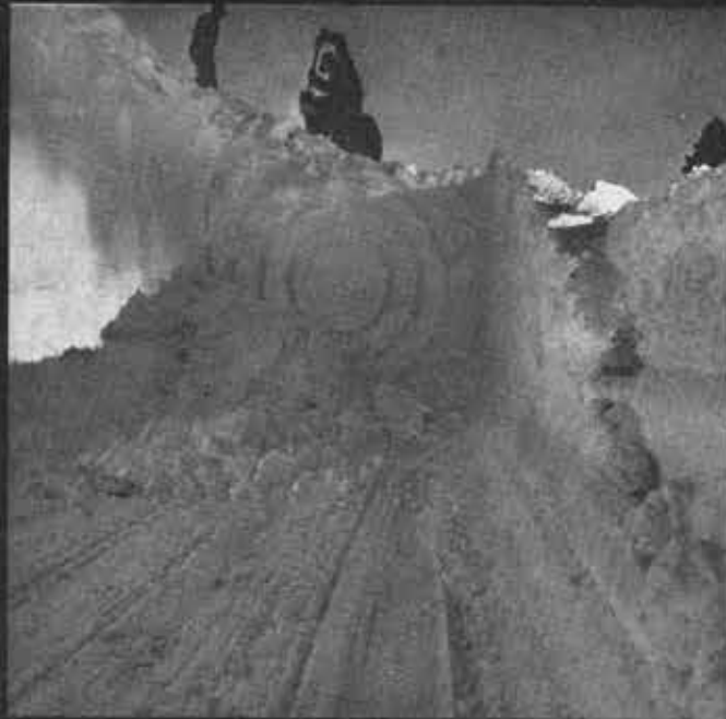
THE ROTARY won its battle with snow, but could not digest rock. At the first crunch, the pilot stopped the wheel and the rotary was backed away so workmen could clear the rocks by hand. After reaching Milepost 321, Rotary OY returned to Osier that night.
