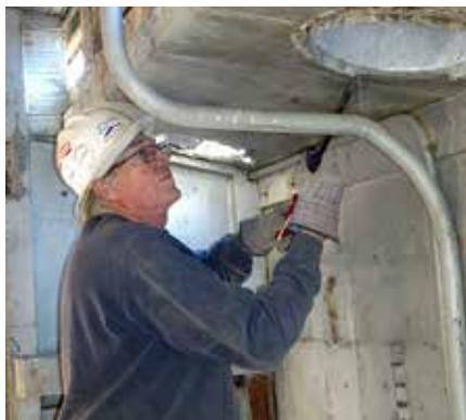
Inspection of the interior for restoration planning.
