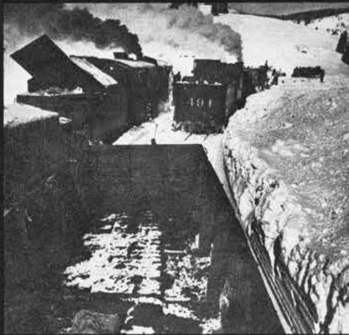
STORY of a snowbound railroad striving to open the line and rescue a marooned locomotive: Rio Grande Rotary OY, which left Alamosa on January 1, pauses in Osier on January 4 after taking three days to plow out the last 5 miles of track immediately to the east.
