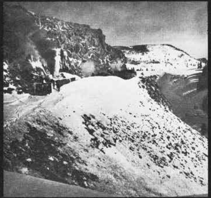
THREE MILES west of Osier, 2-3-2 No. 491 has been stalled in a snowbank since December 29. On January 6, Rotary OY continues the clearing operation, boring out the first cut in a 2-mile stretch of railroad built on a canyon shelf above the Los Pinos River.
