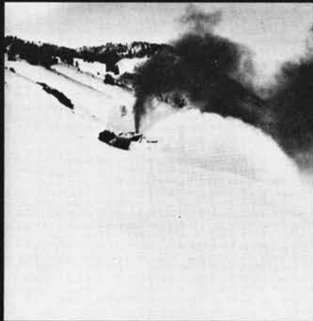
THROWING SNOW almost 200 feet into Los Pinos River canyon, Rotary OY has nearly reached Milepost 321 by midafternoon on January 6. Scene may look peaceful, but the cannonade of exhausts is deafening. Meanwhile, rotary OM reached Cumbres from the west.
