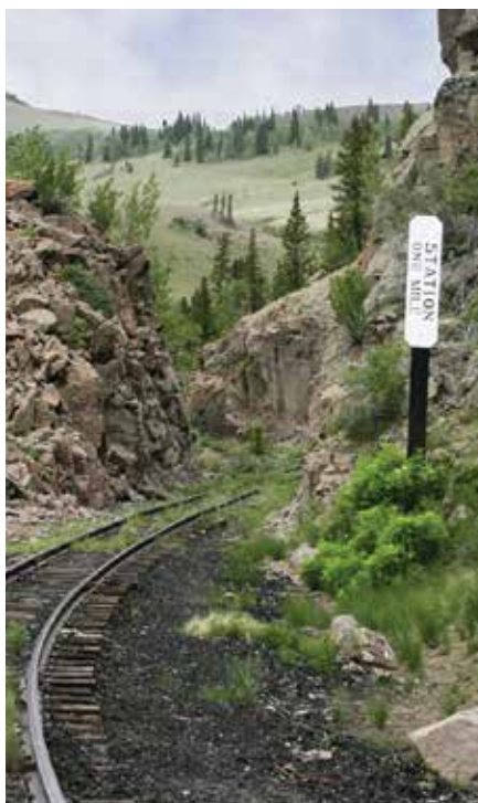
The “Station One Mile” sign was patterned after specifications found in the 1903 edition of the D&RG Standard Signs publication. This recreated sign is located at Mile 317.30, east of Osier. Photo and drawings courtesy Jim Gross
