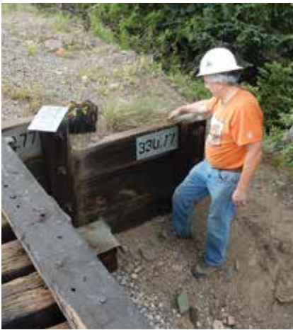
Paul Davenport inspects a bridge plate at MP330 for accuracy.
