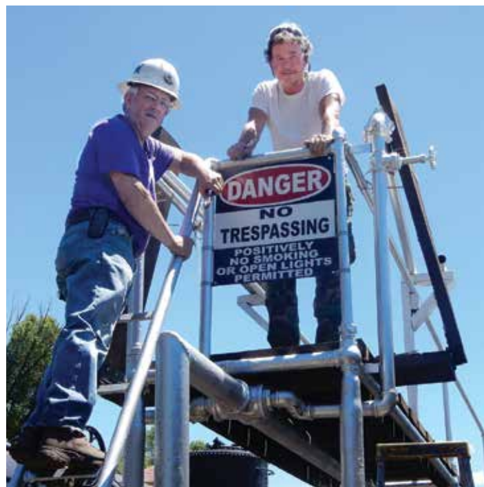
Paul Davenport (L) and Mike Mahoney (R) place a recently completed and historically accurate warning sign on the restored oil loading facility in Chama. Photo by Jim Gross
