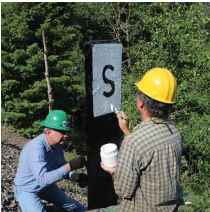
Terry Woolsey (L) and Mike Mahoney (R) repaint a station post along the line. Photo by Paul Davenport
