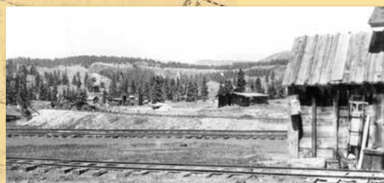
This 1922 photo taken by Charles Lively looks from the corner of the Depot (a portion of the eaves are in the top right corner) looking generally to the north. Note there is no snowshed but it does reveal the windmill, Pump House, cabins and what might have been a single engine house in the distant center that the later-added snowshed was connected to. FCTS RD013-026
