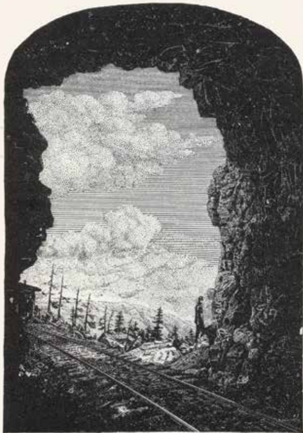
EASTWARD FROM TOLTEC TUNNEL.
