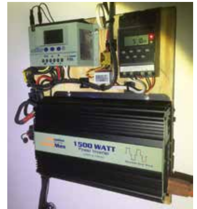
A solar panel and inverter provides power to the Section House and the LED semaphore lights.
