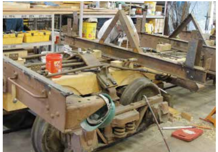
The bolster and cross frame have been reinstalled and the truck has been rolled back in place. The drop door hinges are now being reinstalled with new wood hinge blocks.
