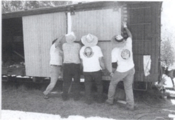
Repair team hanging new side door.
