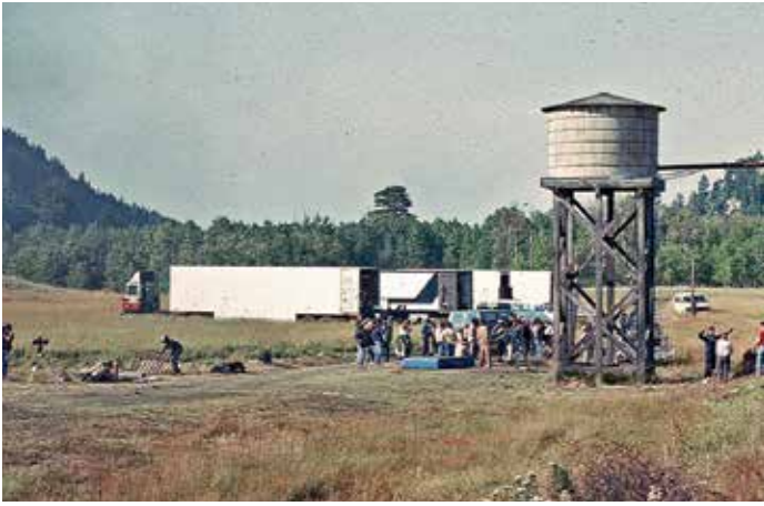
Hollywood set designers constructed a phony water tank and water column at Lobato. Today the tank is gone. The water column still stands.
