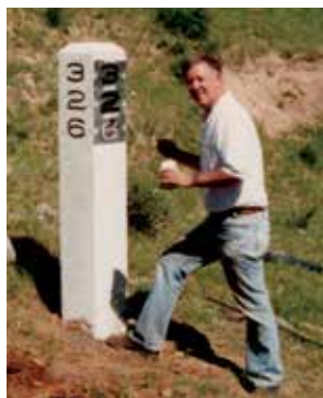
Jim Gross uses the metal C&TS stencil set to complete the installation of MP 326 in 1995.
