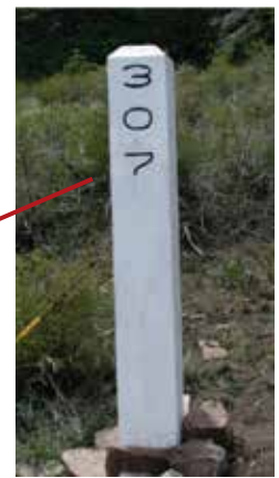
(Left) At some point in the past, MP 307 was replaced, but the style was incorrect and not historic: the mile numbers were painted too low on the post. No similar posts have been found. The MOW Team later replaced the milepost with the correct C&TS design (above).
