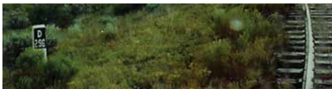
MP 296 as photographed in 1991. The older milepost is now gone.
