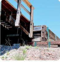
Mileposts can be small metal signs with painted numbers or large wooden posts with the distance in miles to Denver. Mile markers can also be attached directly to a bridge or trestle. The "D" you see on some mileposts stands for Denver.
