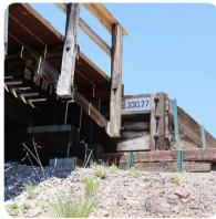
Mileposts can be small metal signs with painted numbers or large wooden posts with the distance in miles to Denver. Mile markers can also be attached directly to a bridge or trestle. The "D" you see on some mileposts stands for Denver.
