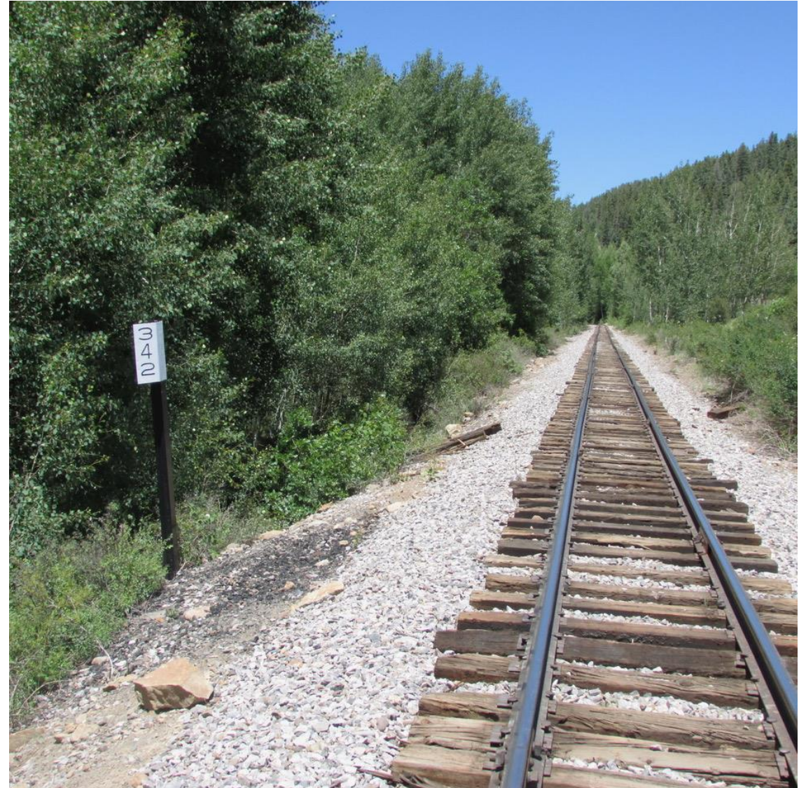
Milepost 342 is an original, all-metal milepost. The post is made from an old rail, the sign from scrap sheet metal bent into a “V” to allow visibility from both directions.
