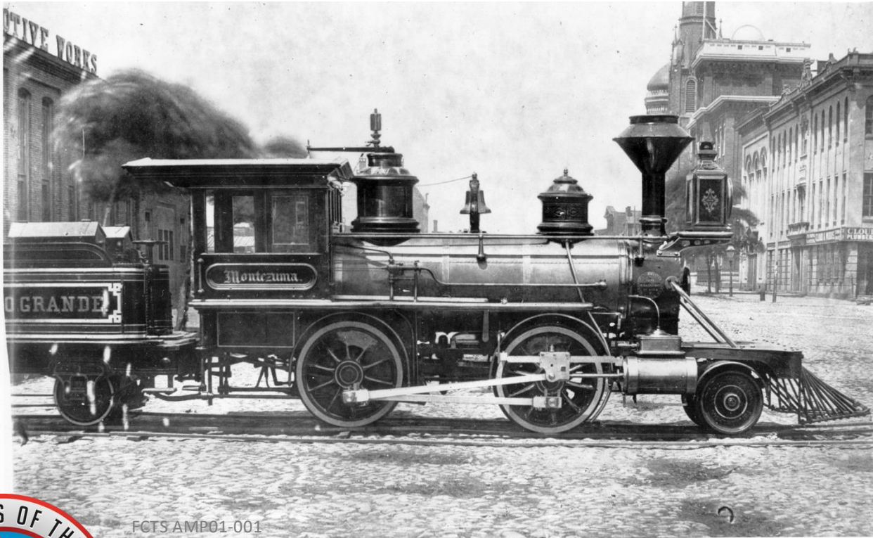
Builder's photo of D&RG #1 "Montezuma. Built in 1871 by Baldwin Locomotive Works. Notice the bell at the center. Taken circa 1871.
