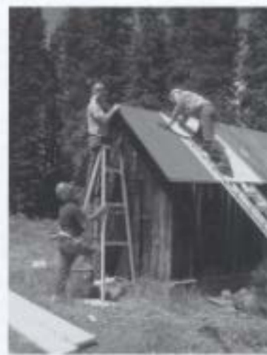
Left to right: Skip Hilgas, Drew Hackmeyer and Jack Warner install roll roofing on the Pump House. (Laura Kammerer)
