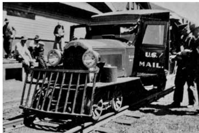
"Motor No. 1" in Rico, Colorado, ca. 1931 FCTS Photo Collection RD169-042
