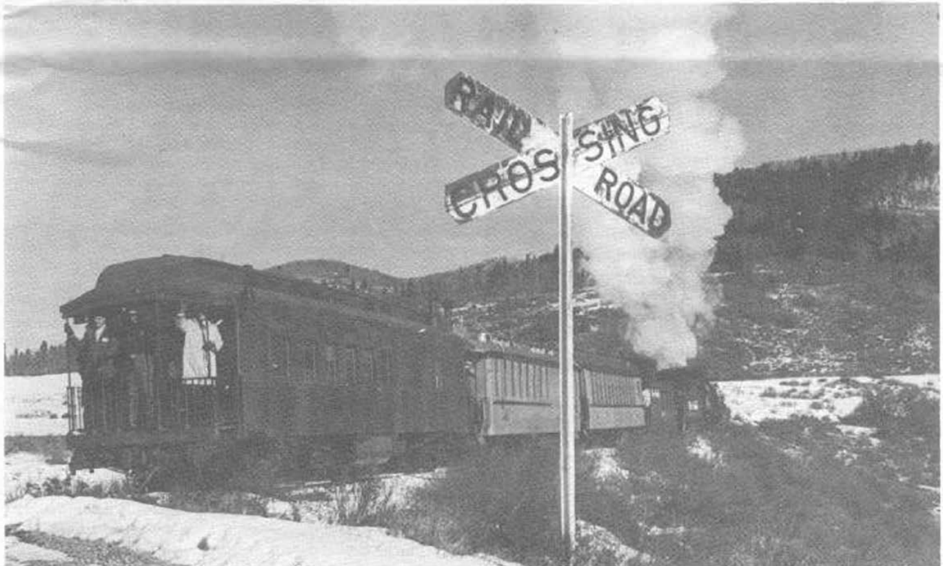
Climbing Cumbres Pass, the National Park Service train crosses state highway 17 near the Colorado-New Mexico border on November 24, 1968. Behind locomotive 483 are caboose 0540, coach 331, combine 212, and business car M-7 (with Union Pacific colors for the film "Butch Cassidy and the Sundance Kid"). Photograph by Ernest Robart.
