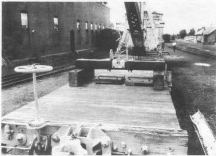
LEFT: Boom tender car with new planking and boom cradle in the Chama yard. The roundhouse and machine shop are to the left. To the right and in the distance is the Chama depot, built in 1899. Photograph by Arthur Nichols.
