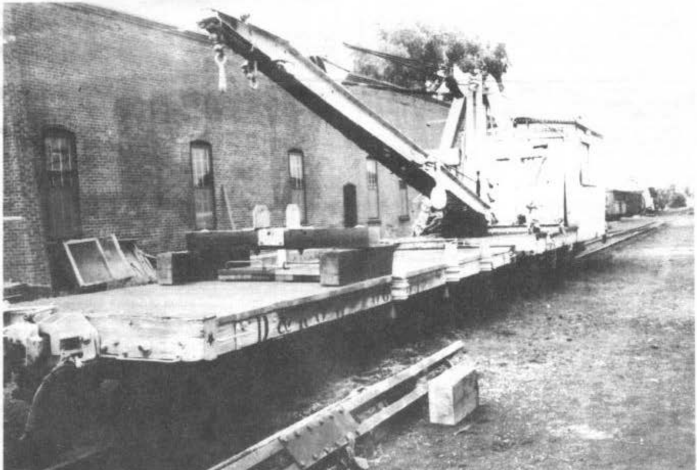
Derrick OP and boom tender car shown in the Chama yard at the end of the July 1990 volunteer work session. Work at the July session included finishing the roof on the derrick house, replacing the many parts removed during the restoration, re-decking the boom tender car and reconstructing the cradle for the boom. The derrick and the boom tender car are ready for painting and lettering. Photograph by William Lock.
