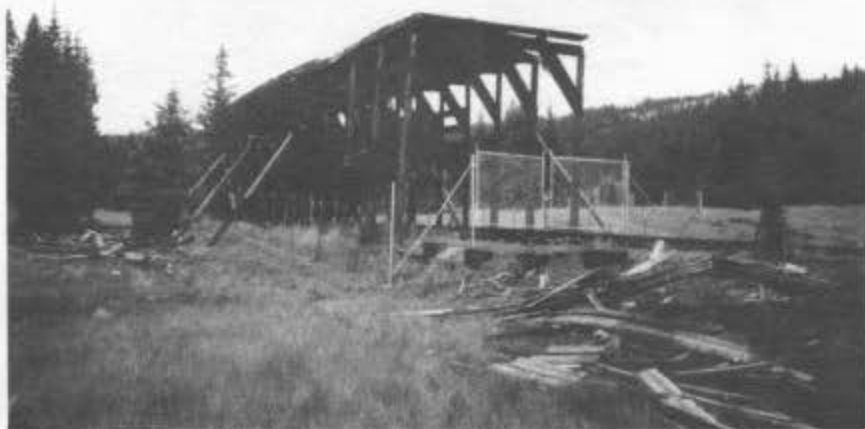
LEFT: The Cumbres snowshed showing the three buttress supports on the west side. Four supports are on the east side. The supports are located at every third post that supports the roof structure.
