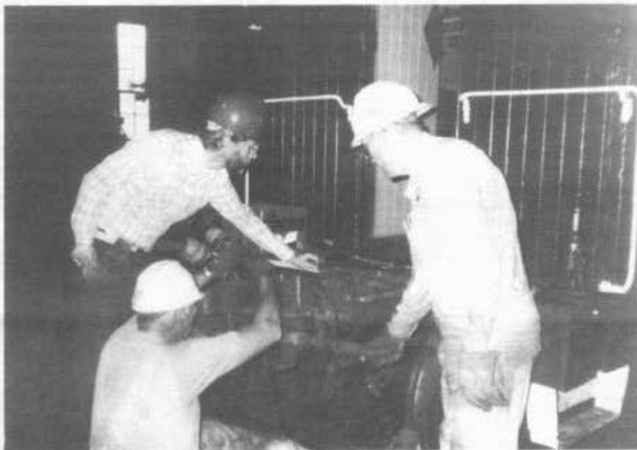
RIGHT: Harry Babcock (kneeling), Roger Breeding (left), and Hawley Seeley working on caboose No. 0503. The old end sill has been removed.
