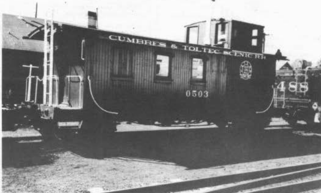
One of the major projects of the August work session: the rehab of historic Caboose No. 0503. The end sill on the near end was totally replaced, the roof was reroofed using modern materials in a historic process, and the inside was refurbished. The caboose is shown here after the photo run-by on Sunday August 19, 1990 during which the Friends simulated a west-bound work extra using restored derrick OP. Photograph by William Lock.
