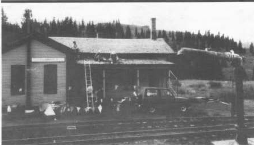
LEFT: Working on the Cumbres section house.
