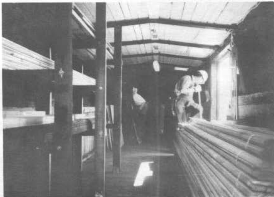
LEFT: Interior view of the Friends new storage car, ex-D&RGW boxcar No. 3686.
