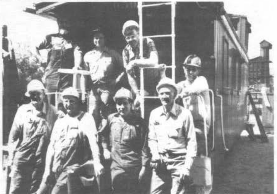
RIGHT: Repair crew for Caboose No. 0503. Left to right, back, are Blake Forbes, Randall Worwag, Marvin Sandmire, and Roger Breeding; front are Hawley Seeley, Harry Babcock (leader), Matt Jameson, and John Carson. The crew removed the old end sill on the A end (opposite the cupola end), fabricated a new one out of oak, and installed and painted it—all in one weekend! Most of the bolts on the old sill were either twisted off or couldn't be removed, so new ones had to be made. John Carson laid out the new end sill, and the other members cut and drilled. John reports that Hawley Seeley and Marvin Sandmire were so creative in finding needed bolts and rods, that "they could probably find palm trees in Alaska."
