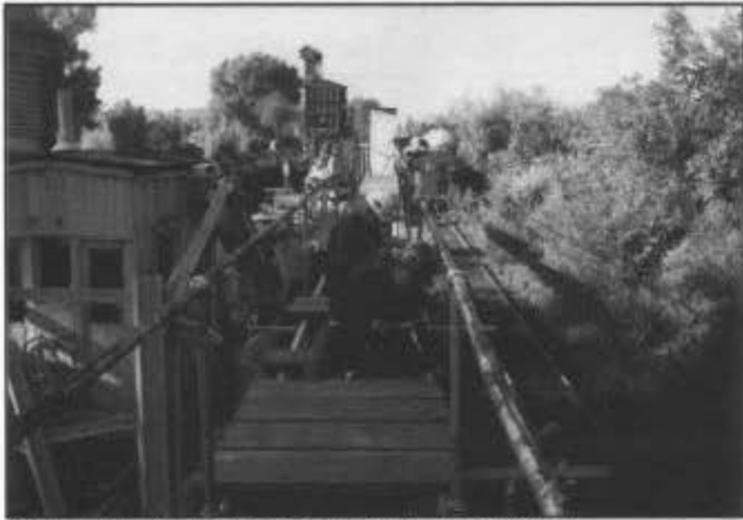
Chama: installing new walkway planks on the oil dock.
