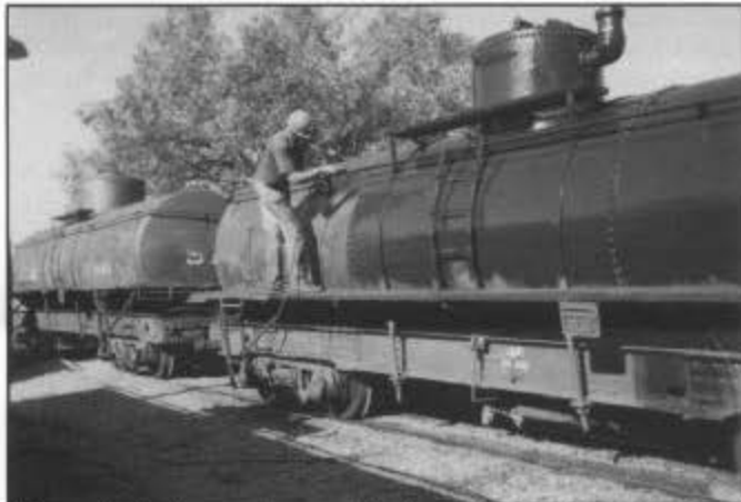
Chama: the tank cars were moved to the south side of the engine house and spray painted.
