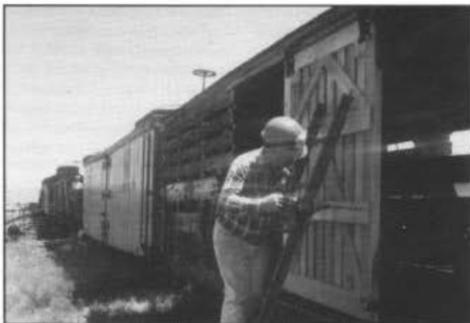
Antonito: installing a new door on stock car no. 5747.
