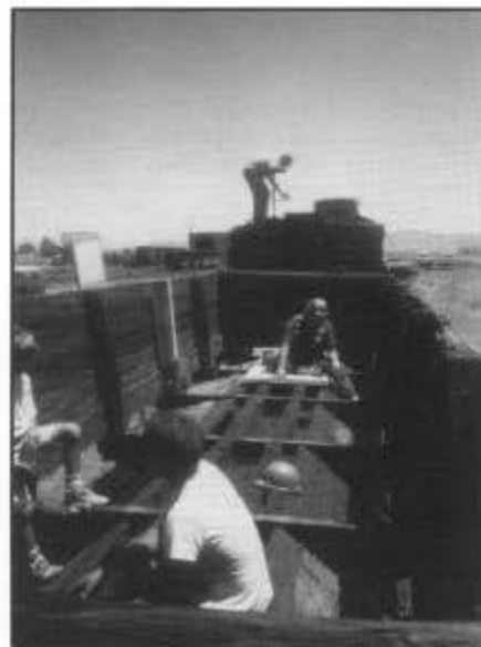
Antonito: replacing rolled flooring in side drop gondola no. 801.
