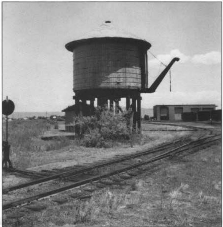
ANTONITO. Looking east, with the engine house in the background. The redwood water tank was constructed in 1977 when the current yard facility was built and is connected to the Antonito town water system. The original (D&RGW) tank in Antonito was located just north of the Rio Grande station in town. August 2, 1992.
