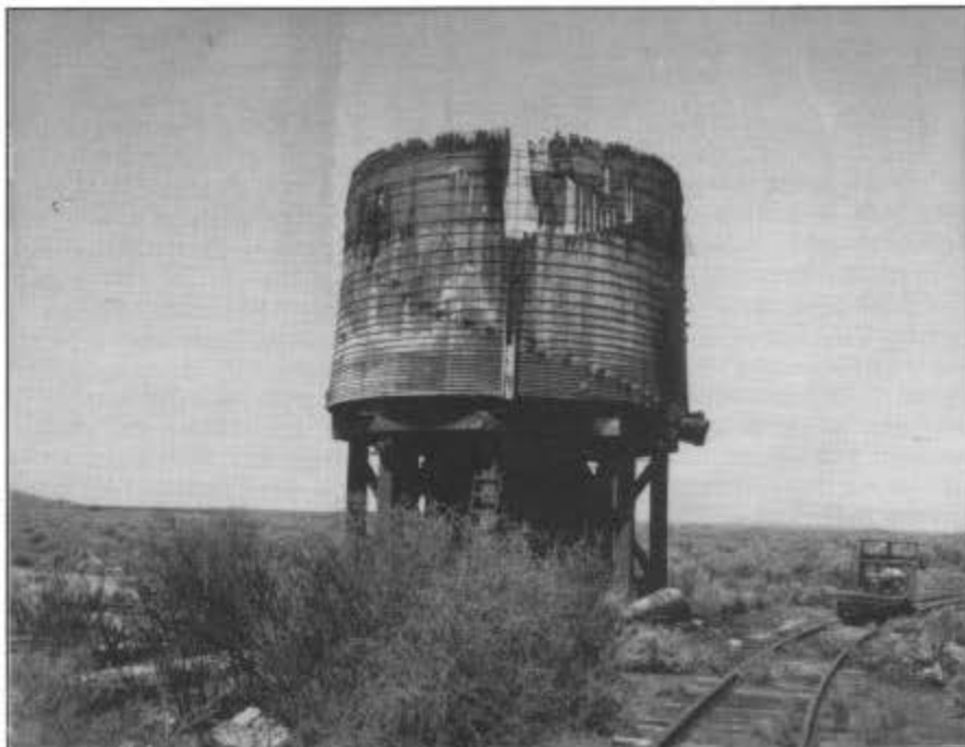
LAVA. This New Mexico State Police photograph (courtesy of Joe C. Johnson) shows the burned out water tank on July 22, 1971. Shortly thereafter, the D&RGW tank at Antonito was dismantled and erected at Lava. During reassembly a small liner was placed inside the tank (approximately 5,000-gallon capacity). A few years ago the pump engine was loaned to the Conejos County Agricultural Museum in La Jara for restoration; the pump itself had disappeared years before. The pipeline from the water tank to the pumphouse is still intact, as is the pumphouse, but the tank is empty and out of service because there is no pump. There are footings for another tank visible just east of the present tank, but whether these footings were for the water tank constructed in 1918 is unknown.
