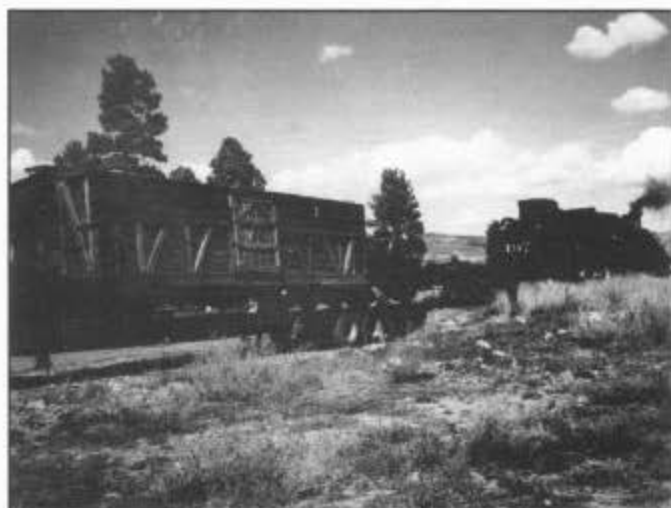
Unloading stock car no. 5600 in Chama at the end of track. The flatbed truck, which brought the car from Alamosa, Colorado, was lined up with the stub end of the track, the stock car was coupled to an idler flat car, and then as locomotive no. 497 inched ahead, no. 5600 was guided on to the rails. John Bush is checking the alignment of the wheels with the rails, while Earl Knoob is in position to signal the engineer. October 14, 1992. Photograph by Carmen Knoob.
