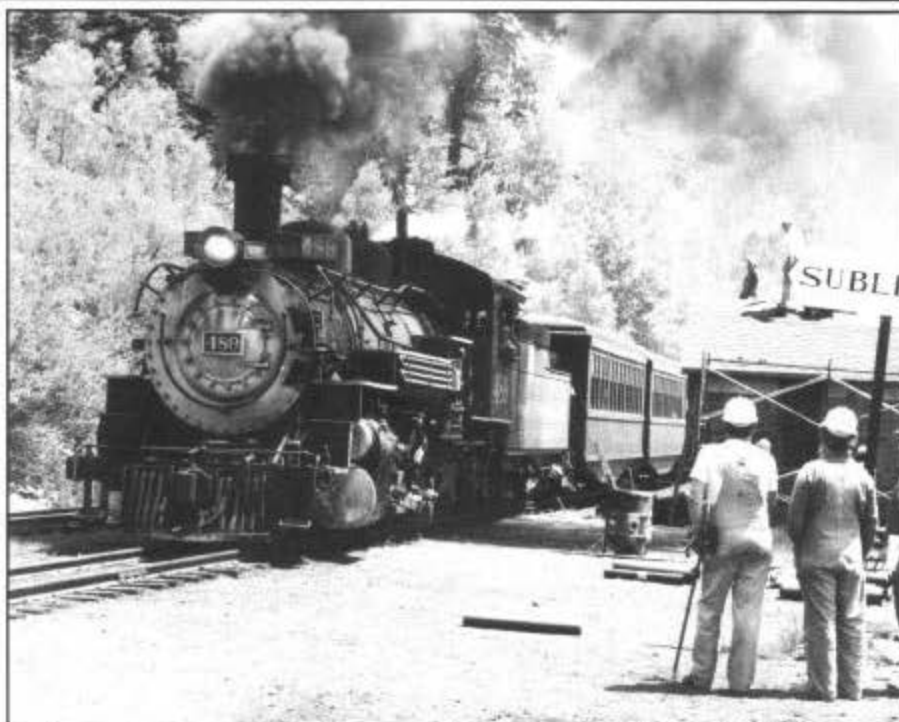
Looking Back—Friends volunteers pause in their work to watch the westbound train passing through Sublette, New Mexico, on the morning of June 11, 1992. Again this summer, volunteers will be carrying out restoration and preservation work on the structures at Sublette, and if hopes are realized, they will finish the three-year restoration with a paint job on the entire ghost town. Photograph by Alfred Judd.
