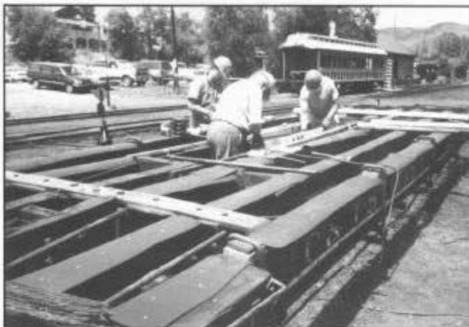
Working on the new floor for a flat car at Chama. In the background a crew from Hollywood is remodeling the Hinman coach for "The Legend of Wyatt Earp." August 1993. Photograph by Art Nichols.
