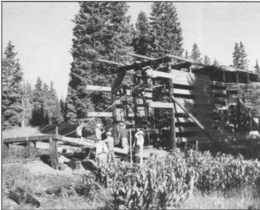
Restoration of the Cumbres snowshed has been one of the ongoing projects of the Friends. Here, in August 1991, volunteers prepare to raise a replacement structure for the first bay. Photograph by Tom Cardin.
