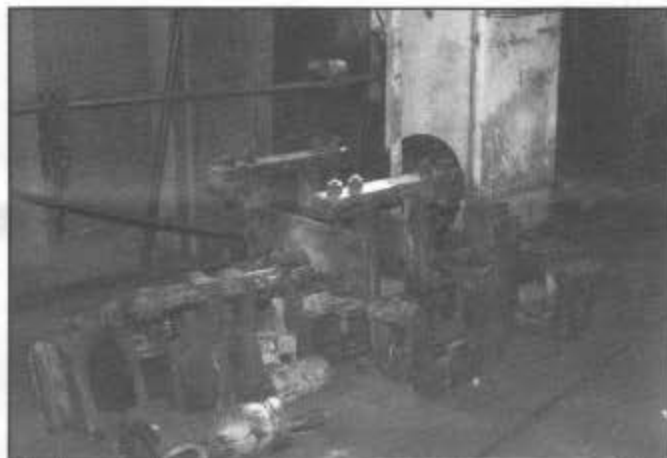
The dismantled trailing truck frame for 463. The frames were fabricated in 1903 for the K-27 class of locomotives, but in 1925 cast frames were used for the K-36 class.
