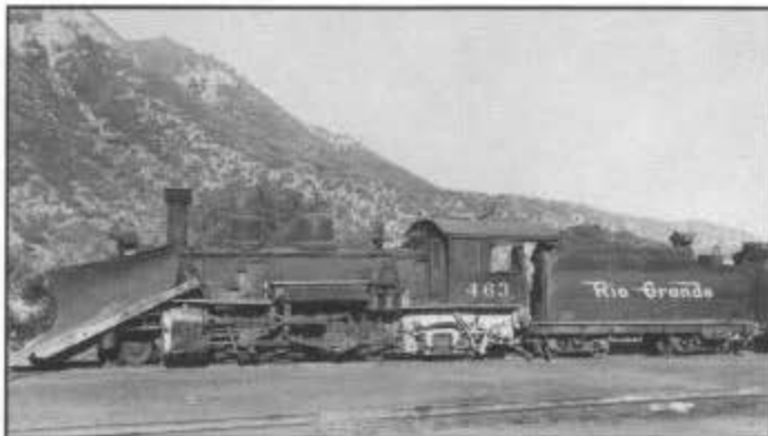
Figure 8. After being equipped with a large wedge plow for bucking snow on the Silverton branch in 1949, engine 463 spent the summer of 1950 in storage waiting for the next winter's snow. The cab windows were covered to prevent snow damage while plowing. Durango, Colorado, June 21, 1950. Stan Kistler Collection.
