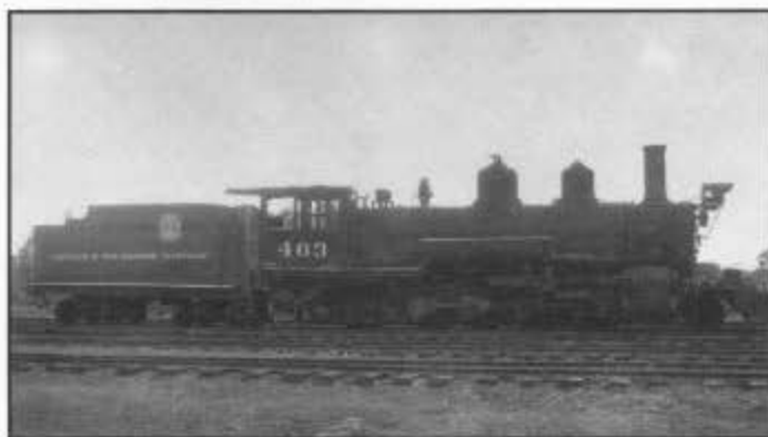
Figure 3. Engine 463 rests in Gunnison, Colorado, on August 31, 1938, after falling through the bridge at Cimarron. The cab roof and the entire left side of the cab is missing. The engine was later hauled to the shop in Salida, where a new cab was built. Robert Graham photo, Tuffard Collection.
