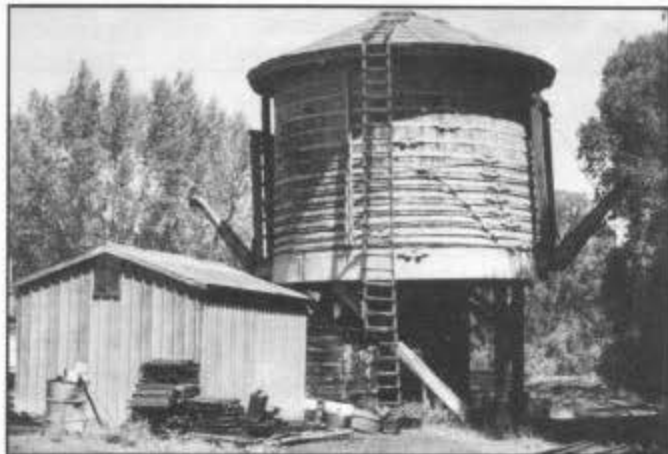
The Chama water tank was built in 1897. Its unique twin water spouts are still in use today. An excellent structure that says, "Model me!" Photograph by Ed Walton, all rights reserved, used with permission.
