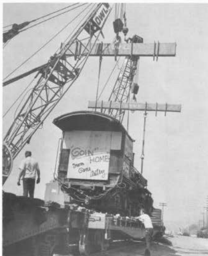
The day after the engine and tender were loaded at Melody Ranch, they were moved to the Southern Pacific's Saugus station for reloading to flat cars. The engine was lowered on to a car that later was found to be insufficient for the engine's weight. Number 463 was then transferred to a heavier flat car at Saugus, but this transfer and repairs to the car later in the Los Angeles yards delayed 463's departure for Antonito by several weeks. February 23, 1972. Joe C. Johnson Collection.
