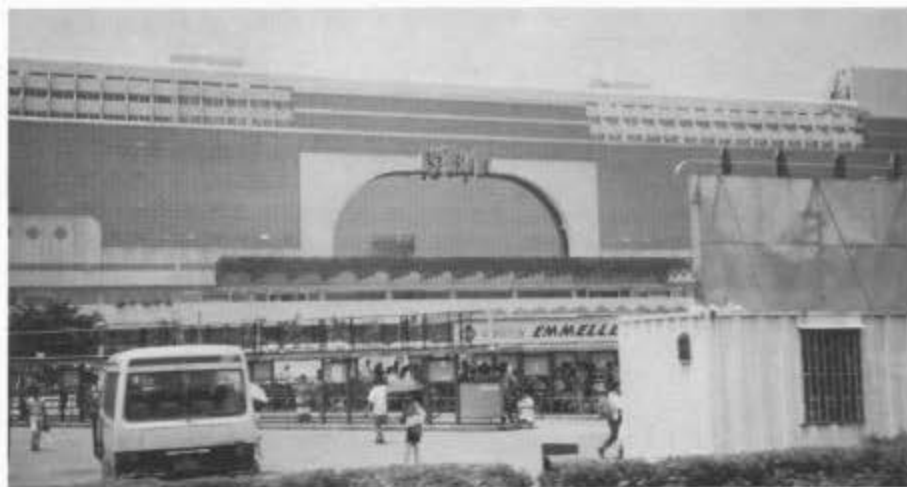
Exterior view of the Shenzhen, China, train station.
