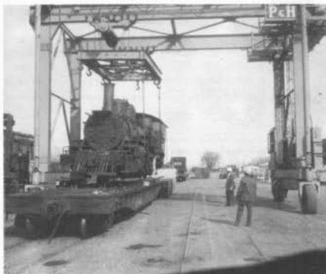
From Los Angeles 463 was shipped through Sacramento, Ogden, Salt Lake City, Grand Junction, Salida, and Pueblo. On March 18, the K-27 arrived in the Denver & Rio Grande Western yards at Alamosa. Shown here, the engine was lifted from the flat car to a flat bed truck, part of which is visible behind the engine. Photograph by Joe C. Johnson.
