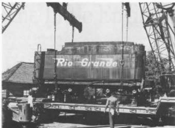
The tender was lowered on to a flat bed truck that brought it to the Saugus, California, station. The tender weighed about 19 tons. February 22, 1972. Tom Klinger Collection.
