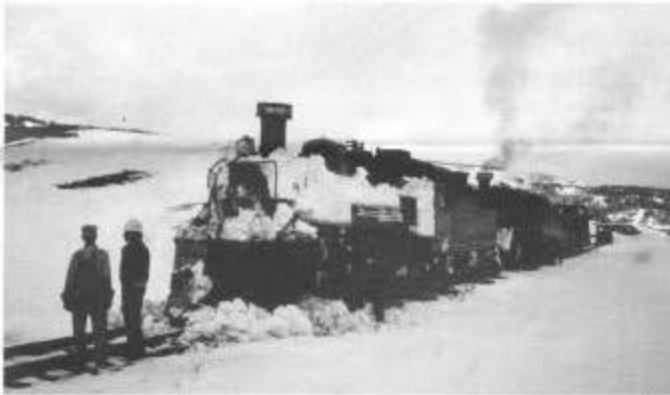
On May 18, after trying unsuccessfully to buck out a seven-foot drift at MP 323.2, the plow outfit (487 and 484) pauses for inspection before returning to Chama. A bulldozer was brought in the next day to clear the line. Note that 487's headlight was removed for plowing to avoid damage. Photograph by Earl Knoob.
