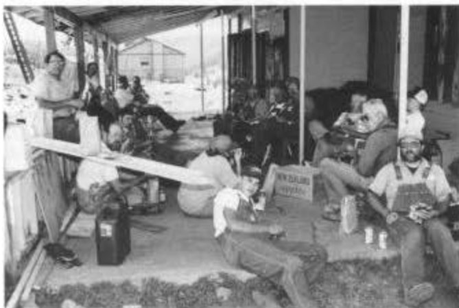
Osier crew dining under the 1970s porch roof of the section house.
