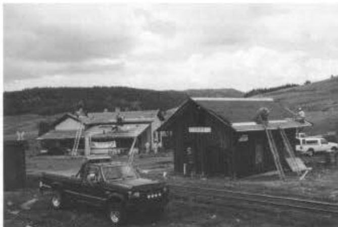
Osier crew installing tar paper underlayment and furring strips on station roof (foreground) and shingling the section house roof.
