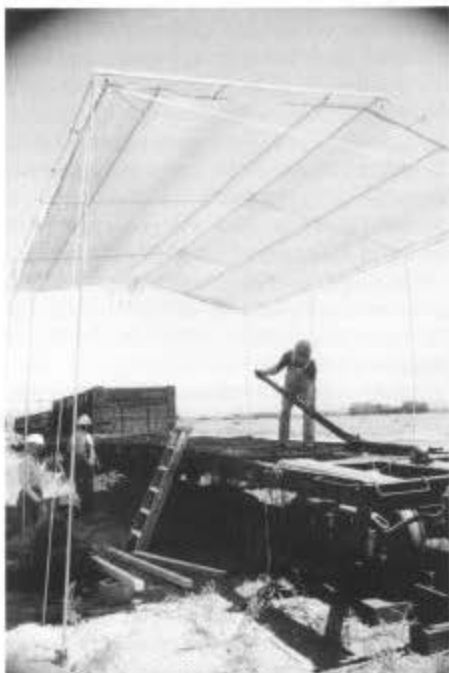
Under the big blue tarp at Antonito, removing old decking from flat car 6627.
