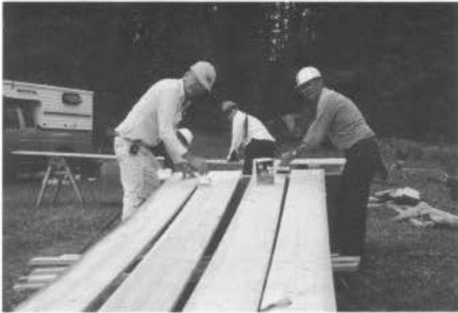
Priming the bottom trim for the car inspector's house at Cumbres.
