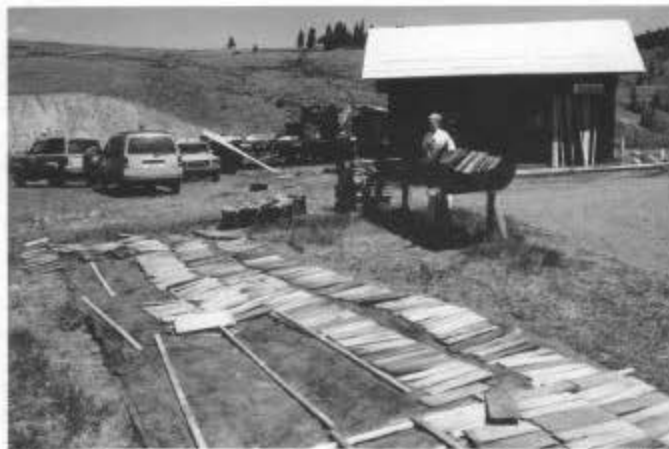
Shingles for the Osier section house roof drying in the sun after being treated with preservative.
