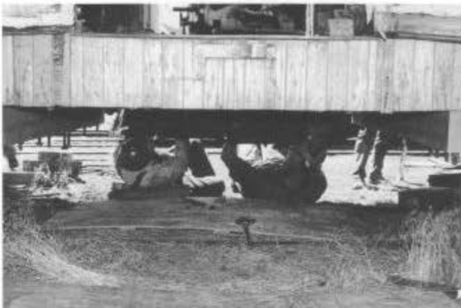
The view most persons get of the crew working on short reefer 55.
