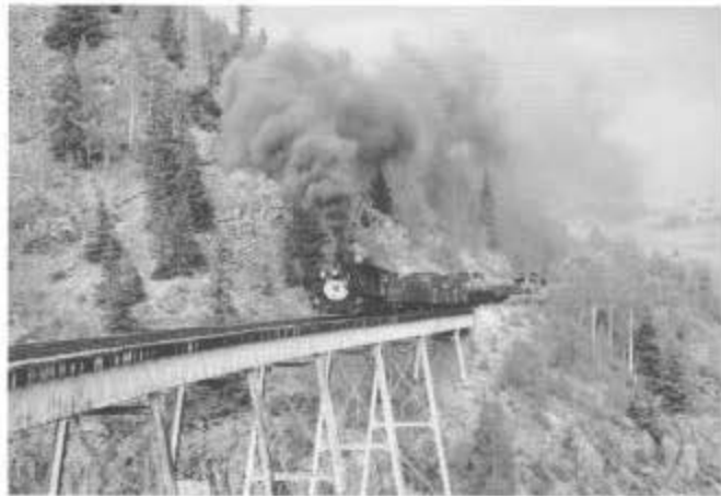
The Friends special train with engine 463 crossing Cascade Trestle, July 29, 1995. Photos by Tom Cardin.
