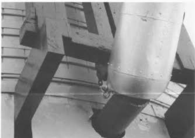
Hinge arrangement of the spout on the face of the water tank. June 1995.
