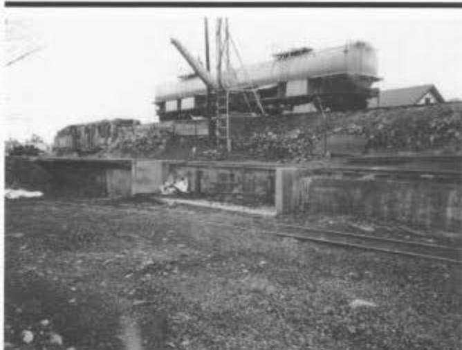
Temporary watering arrangement in the Chama yard on the coal tipple tracks south of the water tank. September 1994.
