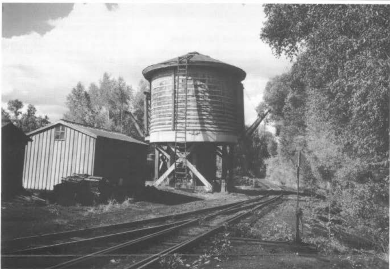
Chama water tank before restoration. September 1994. Photo by George Swain.
