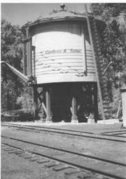
Restored water tank. June 1995.
