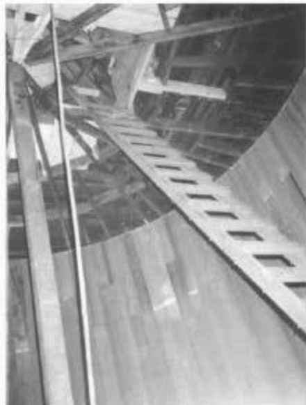
Interior of the new barrel (note the smooth redwood finish). June 1995.
