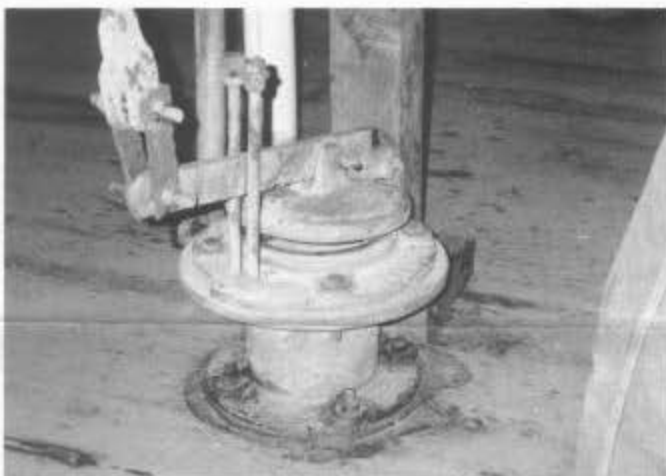
An original valve installed inside the restored barrel. June 1995.
