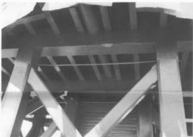
Main beams and chine joists of the restored water tank. June 1995.
