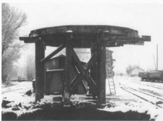
Dismantled water tank on the last weekend of the season. October 15, 1994.
