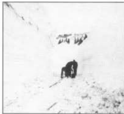
Flanging out ice after backing out the rotary.
