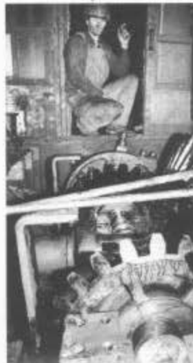
Mark Yates looks over the rotary OY's gears. The broken shaft is shown in the bottom center. This shaft connects the crank flywheel disk to the pinion gear on the left side of the rotary. December 1995.
