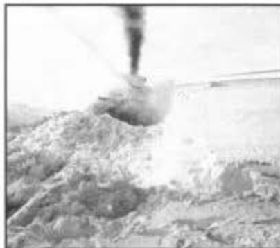
Rotary cutting through a drift east of Osier.
