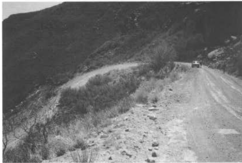
Moro Castle Curve on the Uintah Railway—66 degrees and 7.5 percent grade. Earl Knoob photos.
