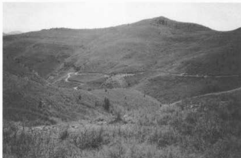
Uintah Railway grade climbing the 7.5 percent grade toward Baxter Pass. Moro Castle Curve is in the distance at the left.
