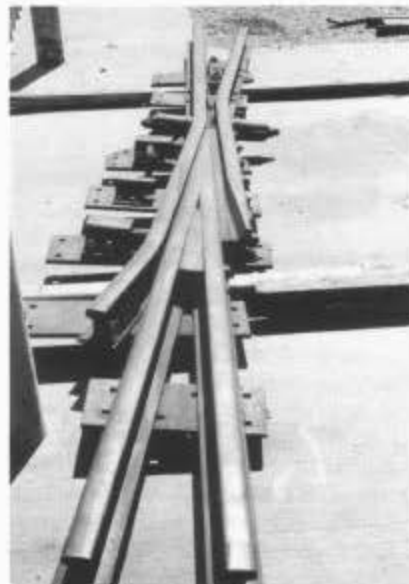
Right-hand switch frog cleaned and ready for painting. Photos by Drake Rice.
