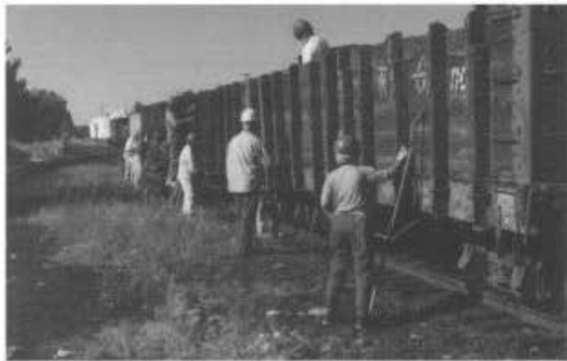
In Chama, the paint crew scrape gondolas before spray painting them. The paint crew gave a second coat to all six sheep cars and painted six other freight cars.
