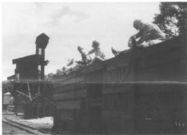
The car repair crew work on a sheep car roof in Chama. They also replaced roofwalks on four boxcars.
