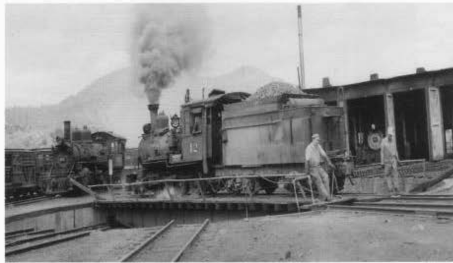
Robert W. Richardson photographed Rio Grande Southern 42 on the Durango Turntable on September 10, 1952. This turntable is similar to the one that was in Chama, immediately north of the brick roundhouse. The D&RGW removed the Chama turntable in 1940. Photo courtesy of the Denver Public Library Western History Collection.
