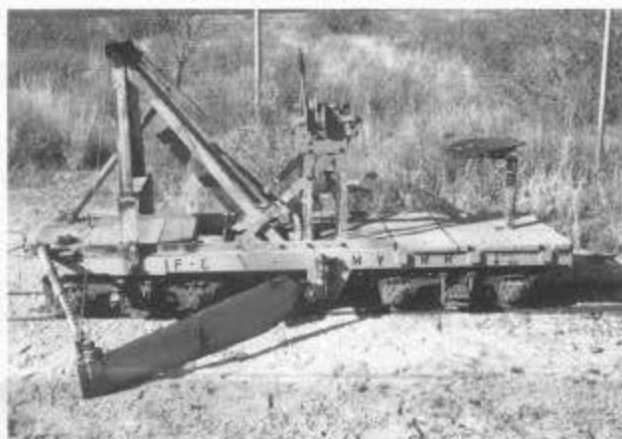
Jordan spreader, a must for preventing washouts.
