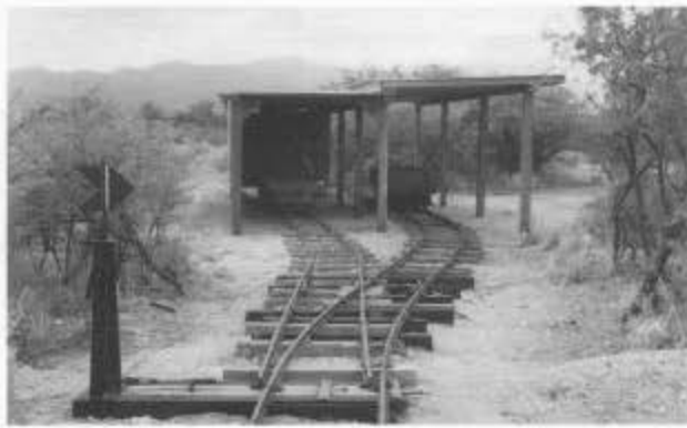
Trackage into the car barn. Note the stub type switch.
