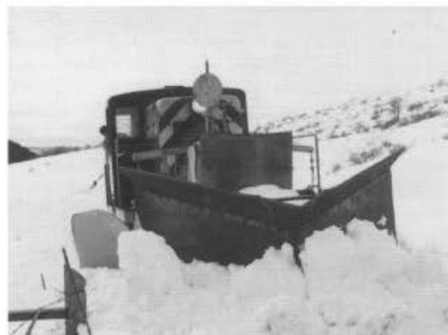
Time to retract the wings on flanger OL at the second crossing of highway 17. Gerald Blea is the engineer, January 14, 1998.
