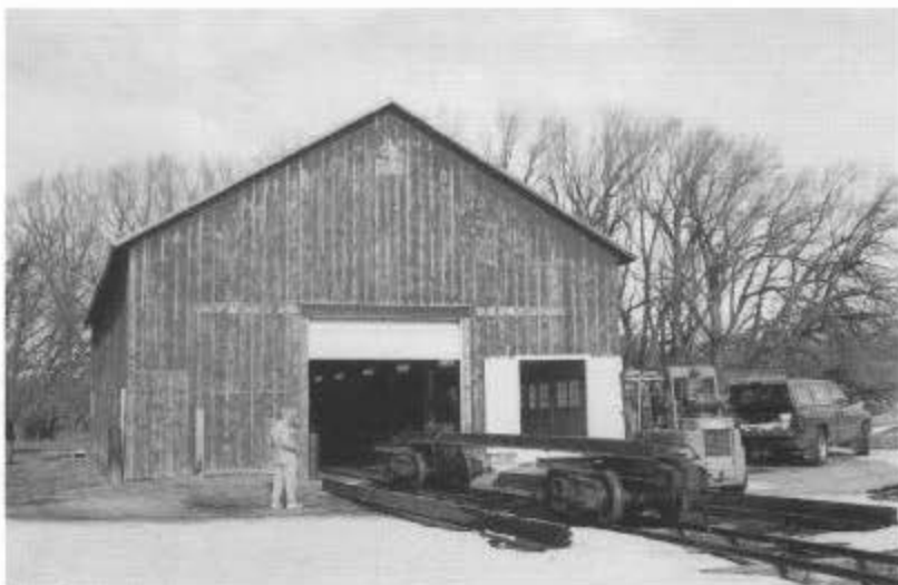
In order to have an enclosed work space, volunteers put down track in front of and inside a nineteenth century dairy barn on museum property, and museum staff installed new light fixtures and electrical outlets. On January 3, 1998, flat car 6200, stripped of all wood and showing the steel center sill, body bolsters, trucks, and couplers, was parked on the track. Art Nichols photo.
