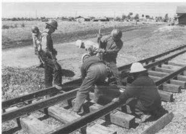
Connecting the three-rail switch to the dual-gauge (three rail) display track in the Antonito yard (session A). This installation is being done for display purposes only as the switch is no longer usable for operation.
