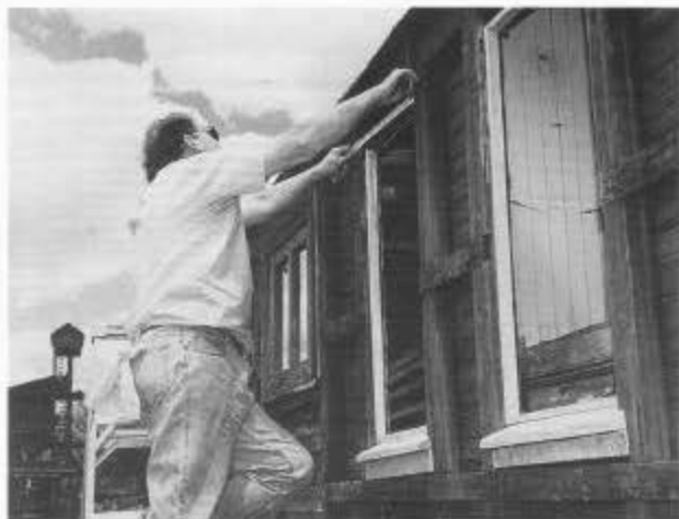
Craig Sutherland measures for replacement window framing on car 053. Note the exposed frame members after the siding has been removed (session A).
