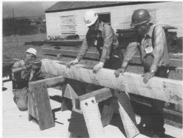
Dave Baughman saws the tenon on the new side sill for flat car 6708 while Drake Rice (left) and Richard Moses steady the sill (session B).
