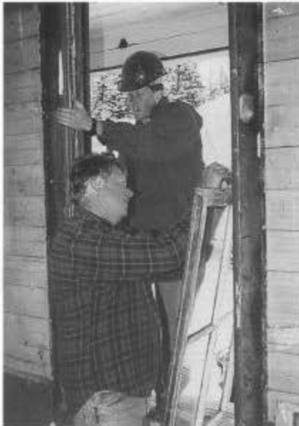
Josh (top) and Al Smucker measure windows in the Cumbres section house (session B). As with the Osier section house, the interior will be restored and upgraded to allow the building to be inhabited during the summer months.
