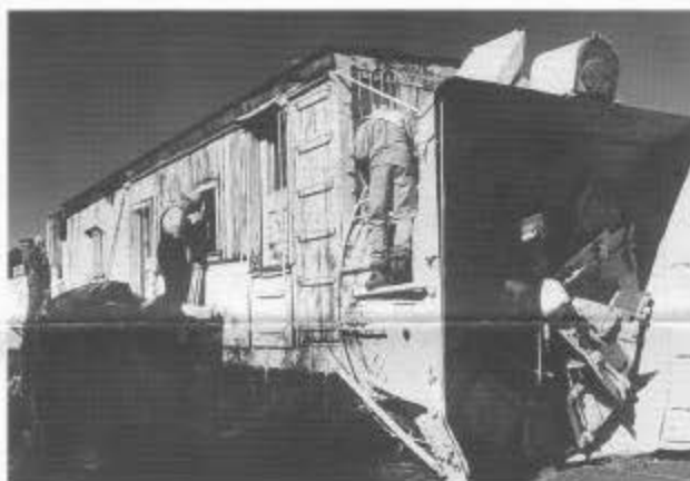
Members of the paint crew scrape old paint from rotary snowplow OM in the Chama yard during session A.
