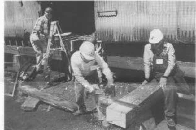
At the corrugated sheet iron building opposite the sand house in the Chama yard, Bill Lock uses a chain saw to cut a loading dock timber while Mike Oestrich steadies the timber (session A). As part of renovating the building for use of one section as a woodworking shop, the volunteers removed the entire deck and replaced it with new material.
