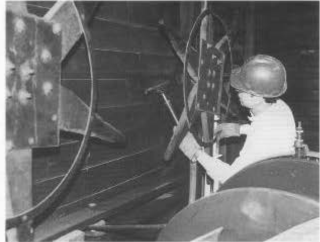
Clyde Putman vacuums the wall of the hoist house. Coal dust has to be removed before paint will adhere to the walls (session A).
