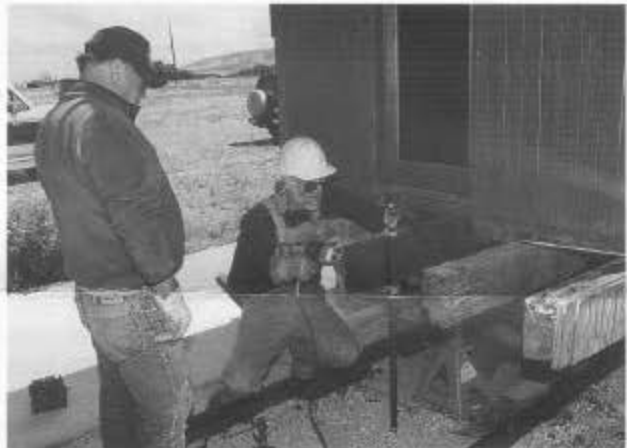
Charles Irvin (left) and Warren Ringer attach steel plates to the frame of caboose 0579 in Antonito (session A). When the frame is reinforced, 0579 could be used in normal operations of the railroad. This car is the only example of a short caboose on the C&TS.
