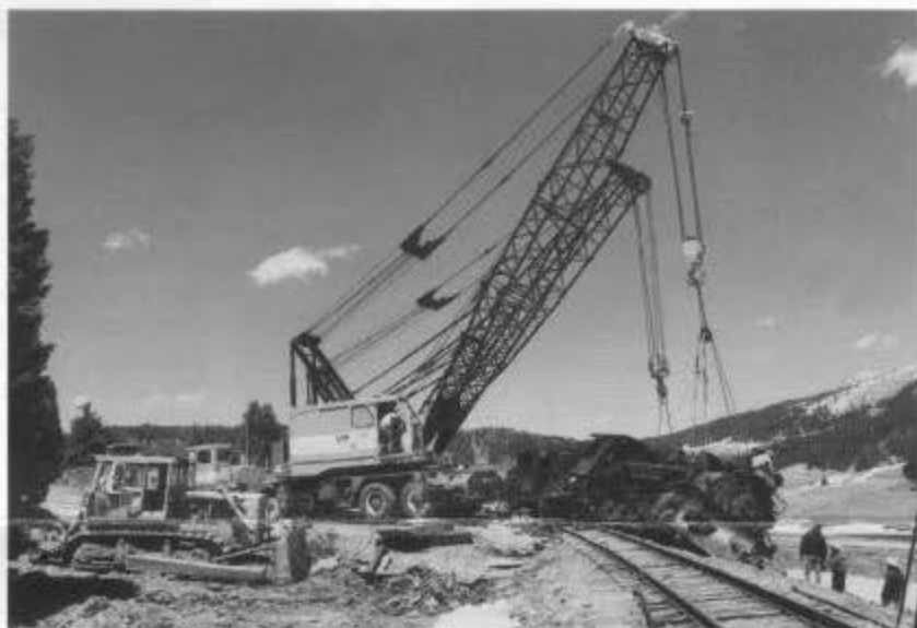
Two, 120-ton cranes in position and ready to lift engine 484 back onto the rails, May 13, 1999. (All photos by Tom Cardin.)
