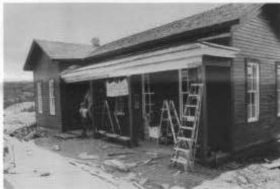
Volunteers completed the new porch roof of the Osier section house (session B). Below, Rich Muth works on window covers for the Cumbres section house. Note the new door and new window frames and sills (session B).
