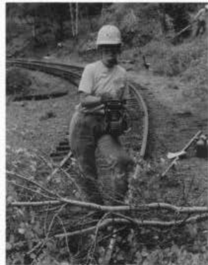
Juanita Smoot thins out trees along the line during session B. Trimming and thinning trees so that a clear area extends 15 feet on each side of the track is done to give the engine crew an unobstructed view down the track and to ensure the safety of the passengers and train crew. (Steve Benezra)
