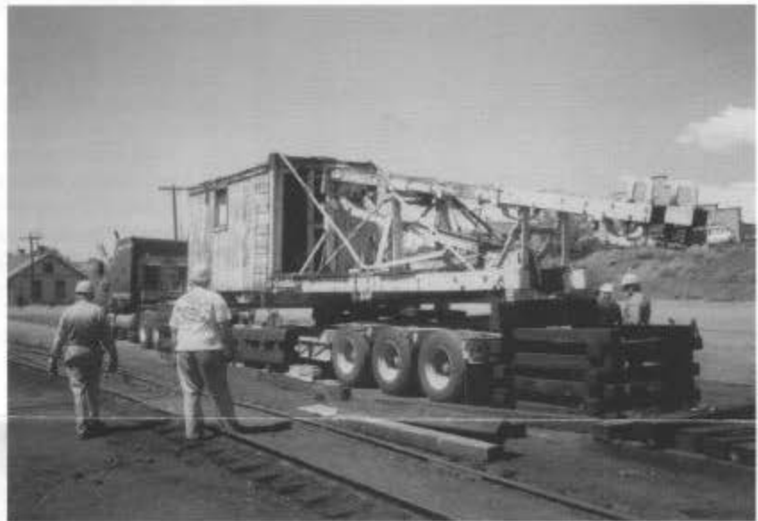
Pile driver OB's superstructure is lowered onto a flat-bed truck in the Chama yard on June 24, 1999. OB's flat car upon which the superstructure rests has been removed. The pile driver, built in 1891, was taken to the Friends' facility at the Western Museum of Mining and Industry at Colorado Springs for restoration. (George Swain)
