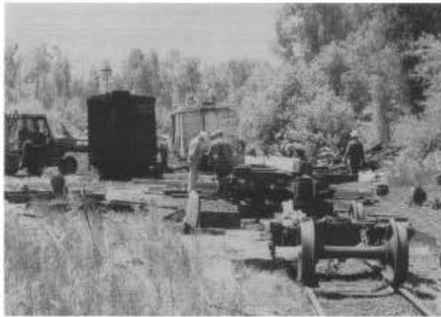
Activity in the east Chama yard, session B. In the foreground, volunteers replace the sills of flat car 6214. In the left background is boxcar 3090, which was cleaned out, and to the right is tool car 04549; volunteers installed a new roof walk, doors and buffer blocks on 04549.
