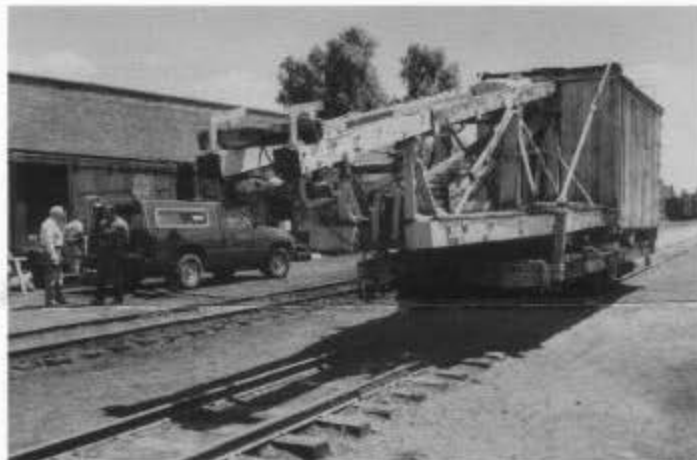
Above, at the beginning of the work sessions, pile driver OB is parked in the Chama yard waiting to be taken for restoration to the Friends' facility at the Western Museum of Mining and Industry at Colorado Springs.
