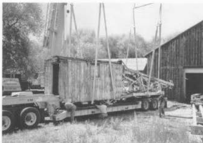
At the Friends' facility at the Western Museum of Mining & Industry, pile driver OB's superstructure (pile driver frame, tower, hoist machinery, and hoist house) being off-loaded after arriving from Chama on June 25, 1999. (Roger Briggs)
