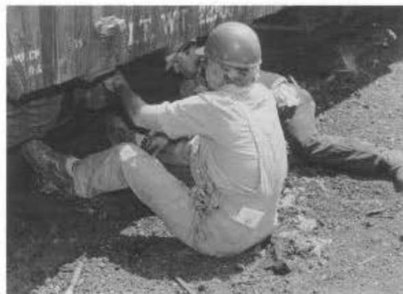
Left, Max Hofman checks bearings on an outfit car in the Chama yard while Art Randall takes notes on the condition of the brake system (session D).
