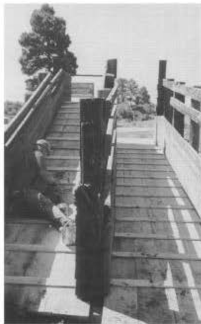
Jim Phelps nails down cleats in one of the ramps in the stock pens at Chama (session C).
