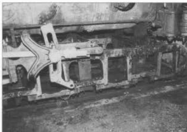
Engine 497 sits high and dry with all the drivers sent to Durango for turning new flange profiles on the tires. Boiler sheeting and insulation have been removed so the thickness of the boiler could be checked by ultrasonics.
