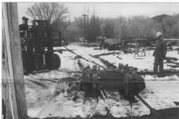
Gerald Blea watches and directs as rebuilt tender trucks are being removed from the enginehouse to make space for another set to be rebuilt.
