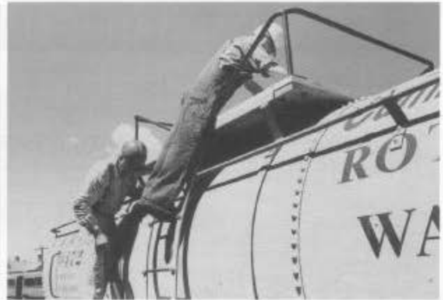
Chuck Templin and Bob Craine working on the new wood decking of Rotary Snowplow OY's water car.
