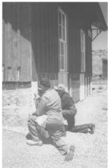
At Osier, John Norcross spray paints under the front porch of the section house (session B). (Below) Ron Carder (front) and Gene Balderston install flashing around the bottom of the old station. The depth of the flashing is the amount the station was raised (session A).
