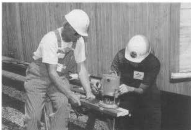
Les Clark (left) steadies and Bob Tully routs siding for the long refrigerator car. The car has 1 x 3-in. siding, but the crew used 1 x 6-in. when the supply ran short. Routing it down the middle retained the look of the smaller boards (session D). (Eric Lundberg)
