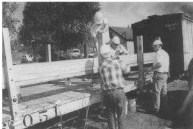
At Chama, the first deck is on the rail and tie car (06051), and now Albert Ruh (foreground), Roy Blizzard (left), Tony Kassin, and Andy Ross work on the second deck and siding (session C). (Tom Cardin)
