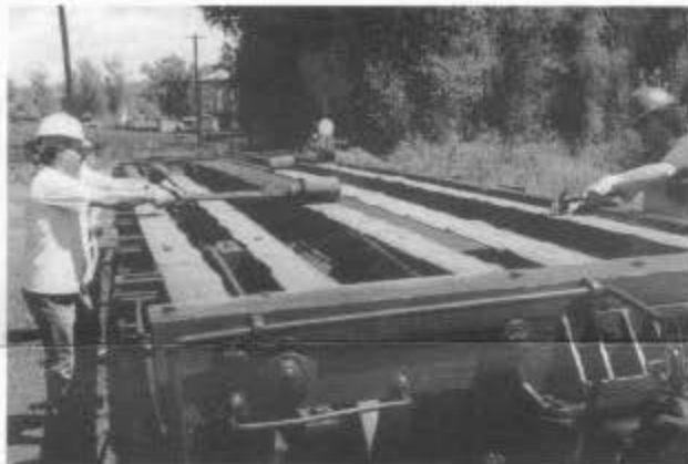
John DeRosa (left) and Benoit Poulin unroll roofing felt to create a moisture barrier between the frame and the deck of rebuilt flat car 6214 (session D). (Tom Cardin)
