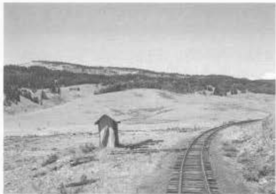
Los Pinos telephone booth at MP 322.95, one of five remaining along the line. A new Friends' project will be the restoration of the booths. (Photo by Art Nichols)
