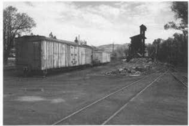
The Chama railyard, looking north, all cleaned up. The turntable components have been moved to the field south and east of the enginehouse, and only a small pile of trash remains to be hauled away.
